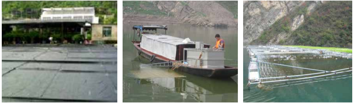
Fig. 2 Treatments of cyanobacterial blooms (Left: shade net; middle: modified clay; right: artificial biofilms and artificial floating islands).
