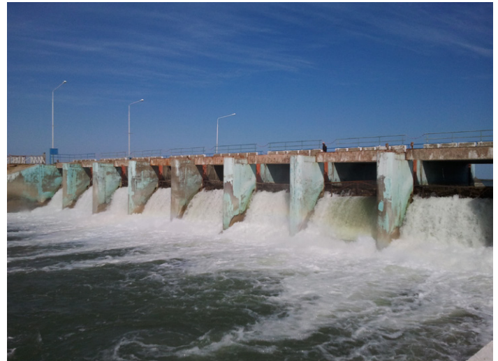
Fig.1. Spillway of Kokaral dam.
