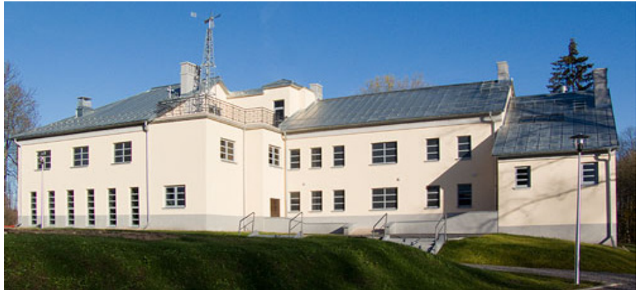
Former Limnological Station on Wigry before II world War and recent Museum of Wigry Lake
