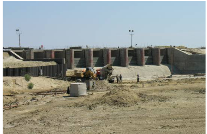
Dike and water spillway under construction, August 24, 2005 (Photo by E. Putnam)
