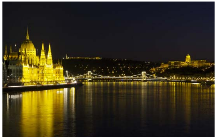
Photo 3. The first stone bridge of Budapest, the so-called Chain Bridge.
