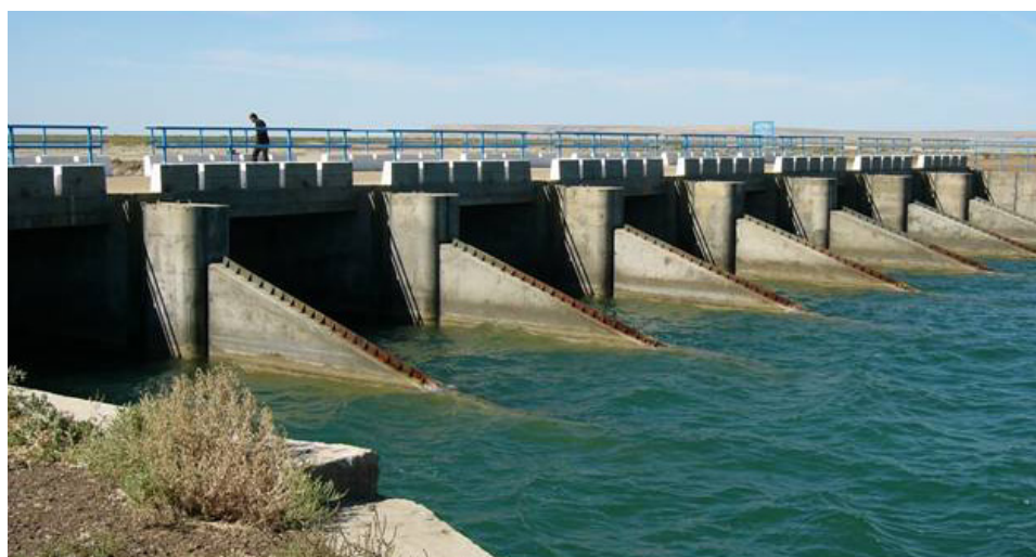
Completed dike and water spillway view from the Small Aral, September 23, 2007(Photo by I. Plotnikov)
