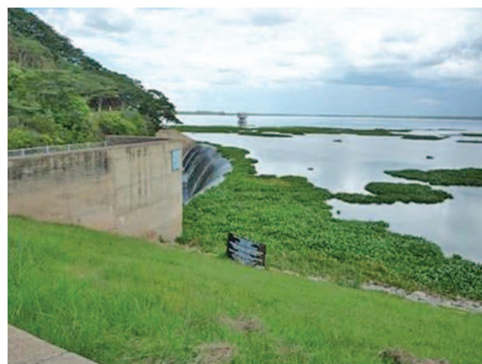
Figure 8. Lake Chivero spillway, showing small amount of water going over the spillway, insufficient to clear the water hyacinth weed.
