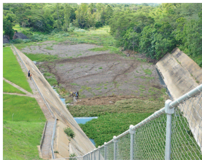
Figure 7. Fishermen working from platform of compacted floating water hyacinth in the L. Chivero spillway channel. The accumulation is due to lack of sufficient flow to clear the channel.
