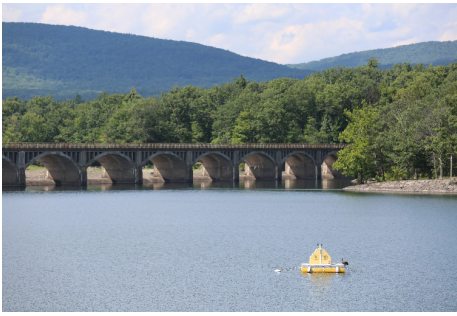
Fig. 3: Ashokan Reservoir dividing weir and a robotic buoy.
